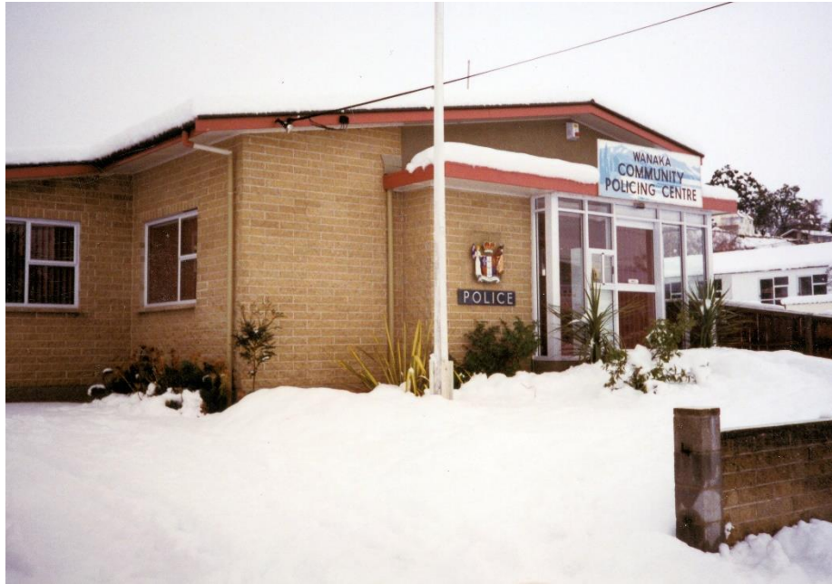
Photograph taken after the 1993 Renovations
